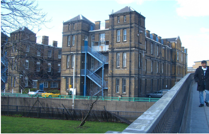
Blick Nr.5:St. Andrews Hospital
